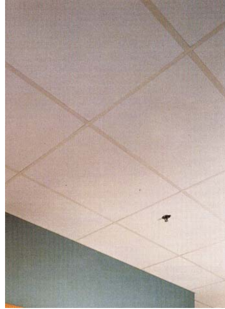
Figure 2 - Food Store Suspended Ceiling
